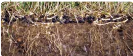
View of the GreenArmor System, demonstrating extensive root development within and below the reinforcing matrix.
